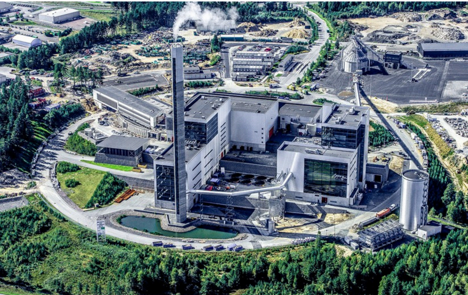
MSW-fired Waste-to-Energy plant powered by Kanadevia Inova (HZI) Steinmüller technology
