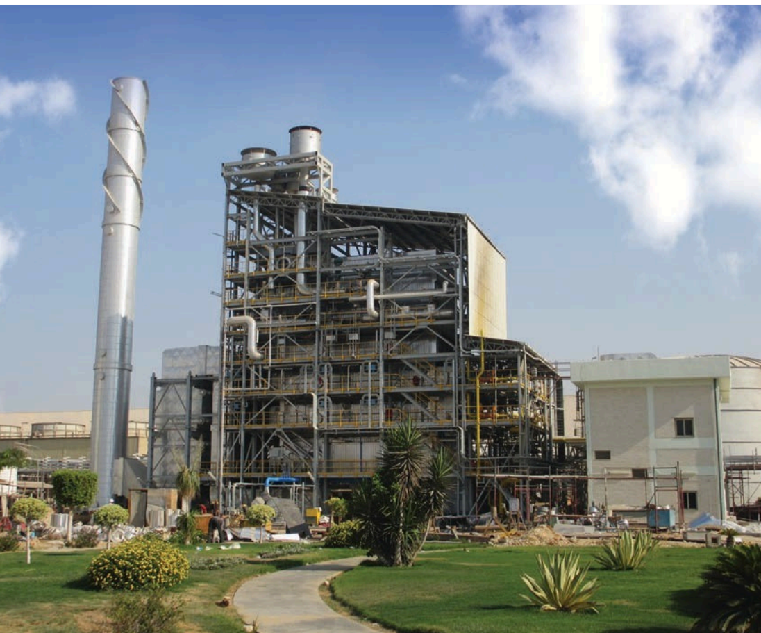
1 unit of 175 TPH, 115 kg/cm 2 (g), 510°C natural gas, diesel fired boiler
