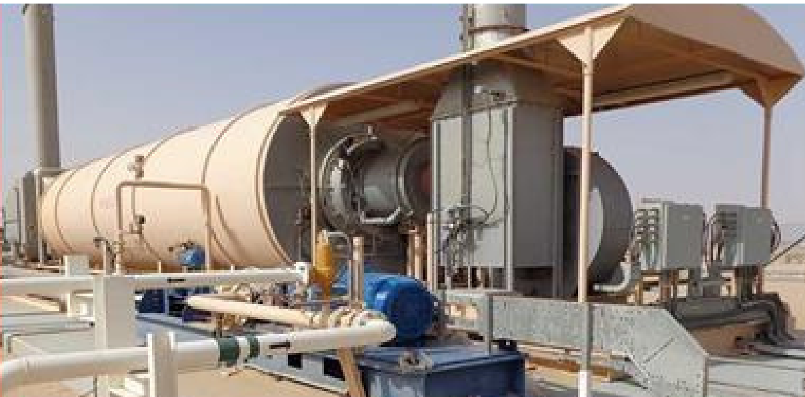
Once-Through Steam Generator Installation
