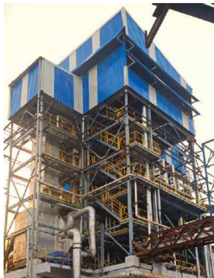
The 15 TPH Flexisource™ boiler installed in West India
